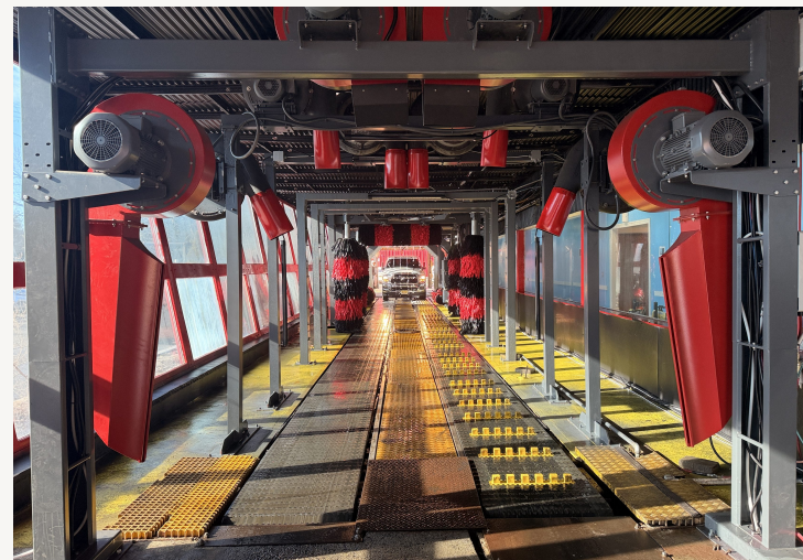
A conveyor tunnel in service. Dryer blowers on the near gantry, brushes and a vehicle further down the line, with the conveyor track set into the floor between the guide rails.
